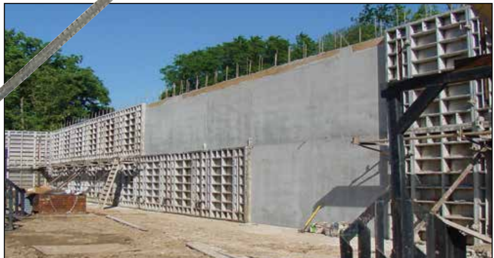
Big Panels stacked to achieve a 16' wall on a commercial project.
