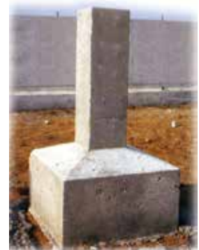
Column and footing design in one placement.
