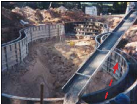
PLACING CONCRETE
